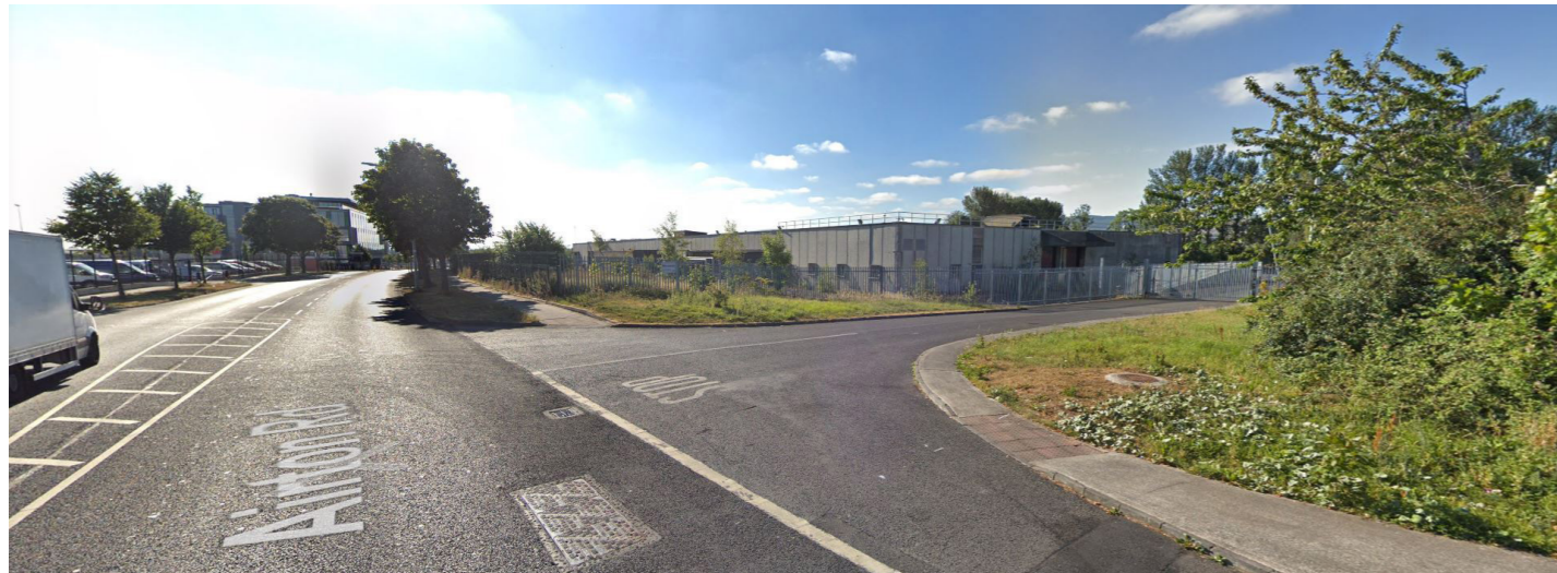
SITE ACCESS OFF AIRTON ROAD
