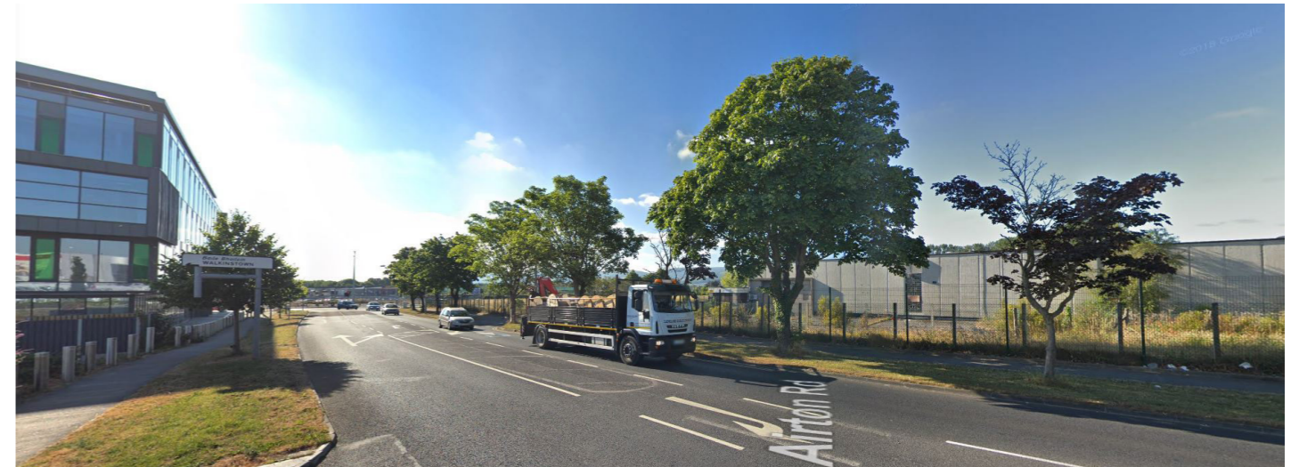
VIEW FROM AIRTON ROAD LOOKING EAST TOWARDS INTERSECTION WITH GREENHILLS ROAD
