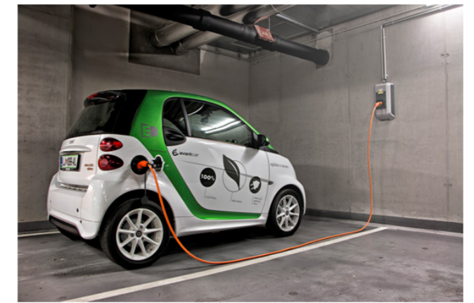
ELECTRICAL CHARGING POINT
