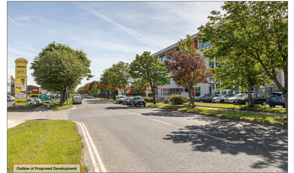
VIEW - 03 FROM AIRTON ROAD LOOKING EAST
